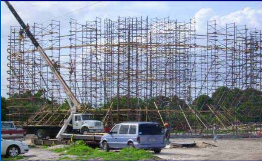
3 MG Storage Tank Construction
